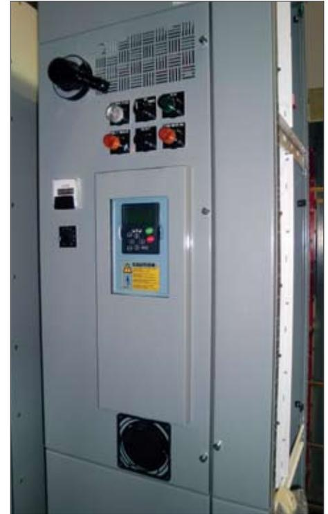
*Variable frequency drives can be installed within a motor control center as this Westinghouse Type W sample shows. A waste water treatment plant in Arizona had limited space and required a custom engineered solution utilizing a 'bubble' door.*
