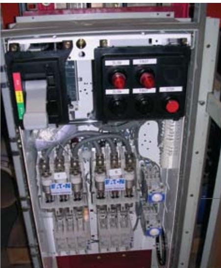
This Westinghouse Five-Star MCC bucket was retrofitted with a two speed, two winding, vacuum starter.
