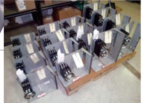
*These GE 8000 units needed a quick change to feeder buckets to accommodate new equipment.*
