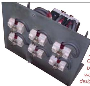
A very old GE MCC bucket was custom designed to accommodate dual stabs for increased amperage.
