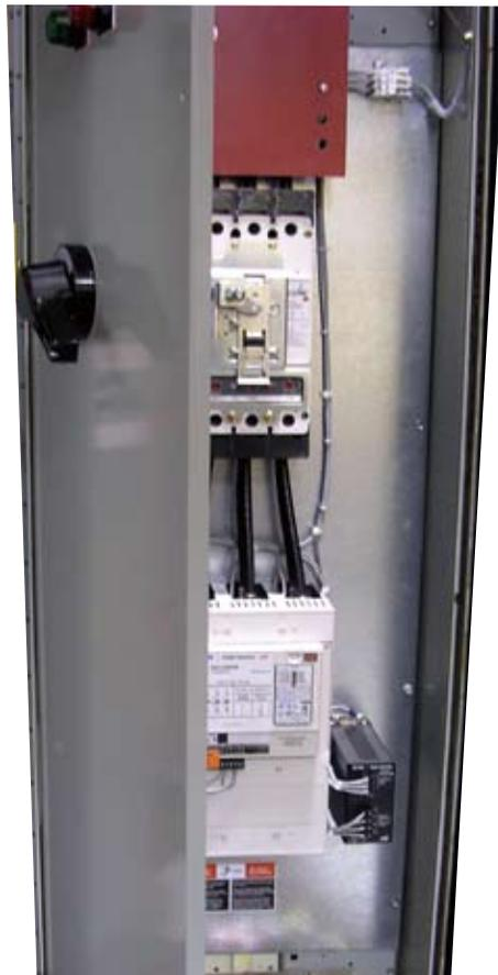
*This soft-start retrofit for a 250 HP motor offers long term cost savings and reduced a tripping nuisance. Utilizing a custom backpanel approach the design reduced installation costs and minimized downtime, compared to a new MCC, and improved reliability.*
