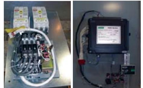
*A Westinghouse Type W MCC at a large refinery was retrofitted with a new ASCO Automatic Transfer Switch. Retrofitting with a new digital control Automatic Transfer Switch will restore the critical transfer of power function in an emergency situation.*
